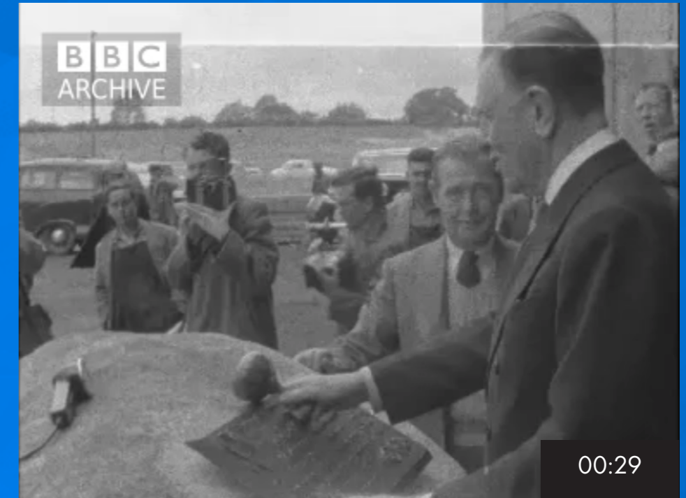
Lord Wakehurst, the Governor of Northern Ireland laying the foundation stone of the new general hospital. From: "News: Governor of Northern Ireland Lays Foundation Stone" (1956)
