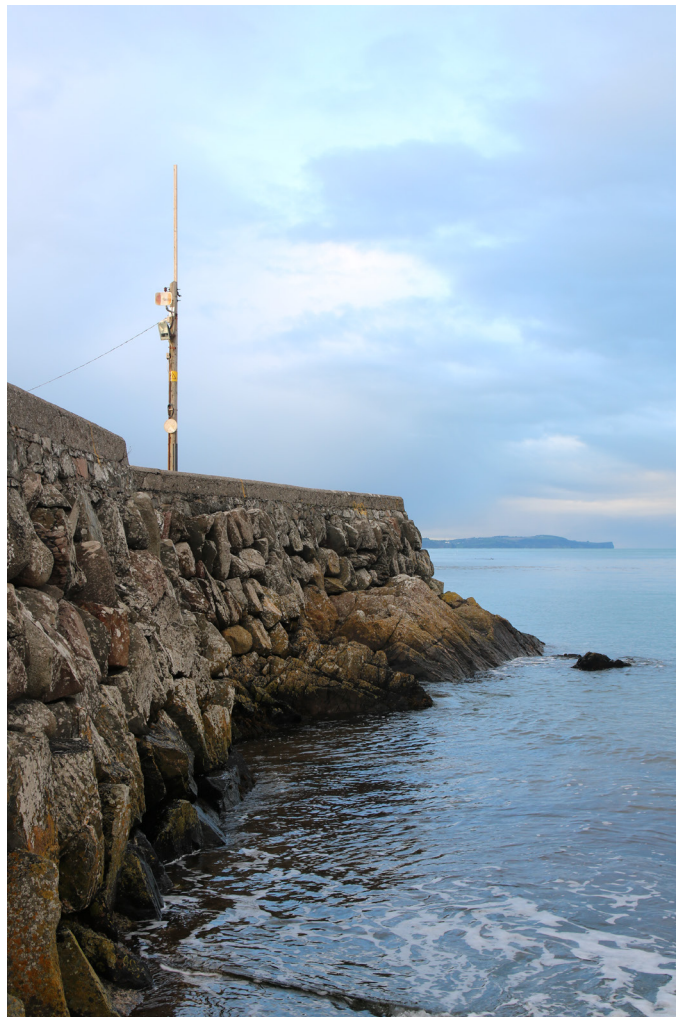
"Seawall at slipway"
