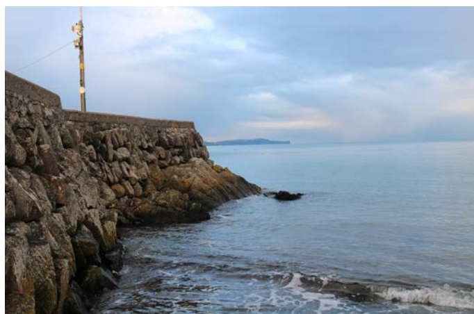
"Seawall at slipway"
