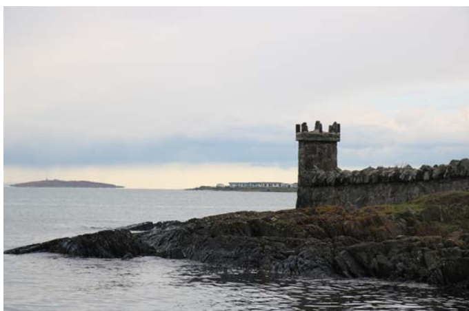
"Shore at seawall 1"
