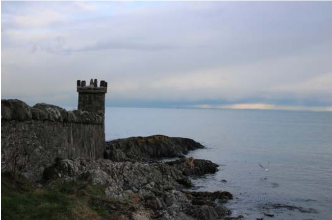
"Shore at seawall 3"
